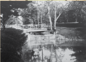
1. Pictured here and drawn on this 1876 map, a pond occupied part of what is now Sherwood Gardens.
